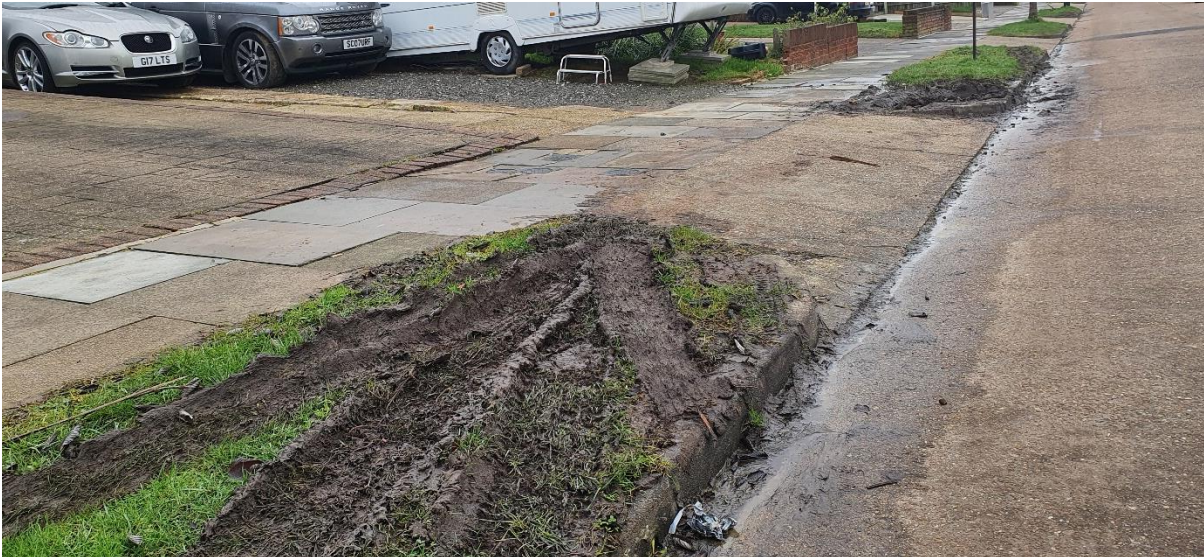
Figure 14 – example of damage to grass verges
